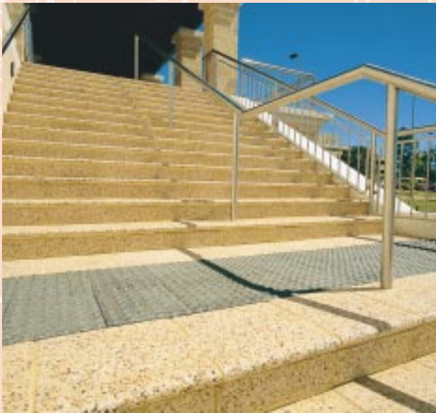
City of Joondalup Cultural Centre - exposed aggregate, tactile modules and bullnose stair treads installed for safety and durability.
