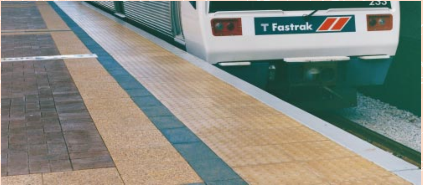
Perth's Northern Suburbs Transit system - exposed aggregate and tactile pavers used for durability and safety.
