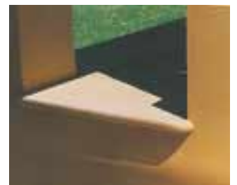
Radius bullnoses used in walls.
