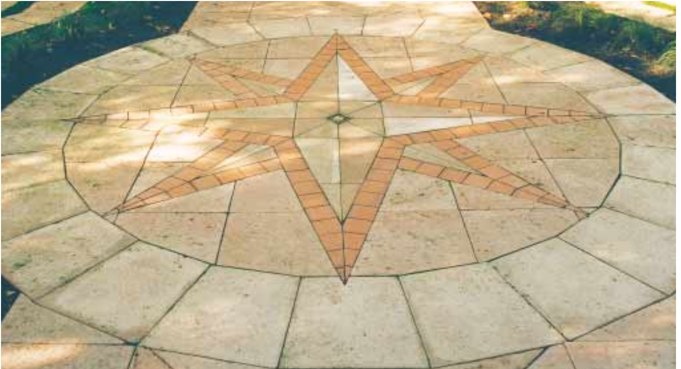
Salmonback paving with Limestone Reef header and star pattern using Tuscan, Salmonback and Limestone Quarry inlays.
