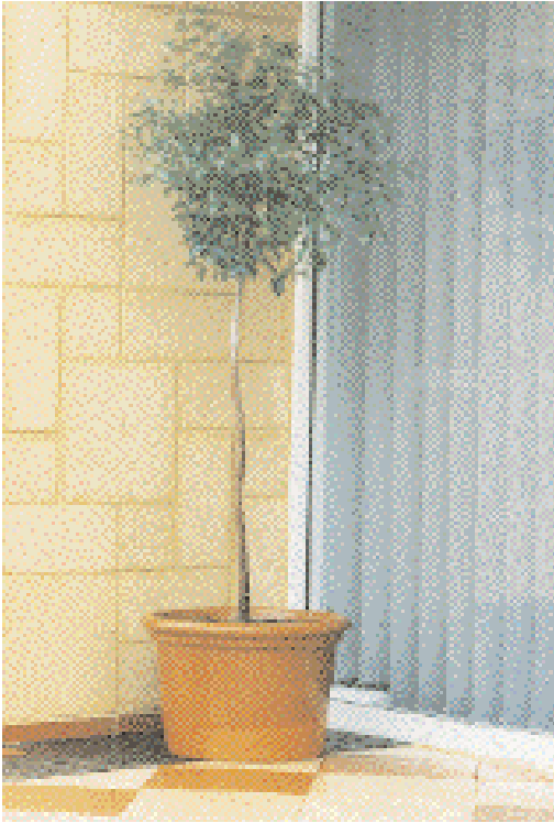
External wall with Limestone cladding in random pattern.
