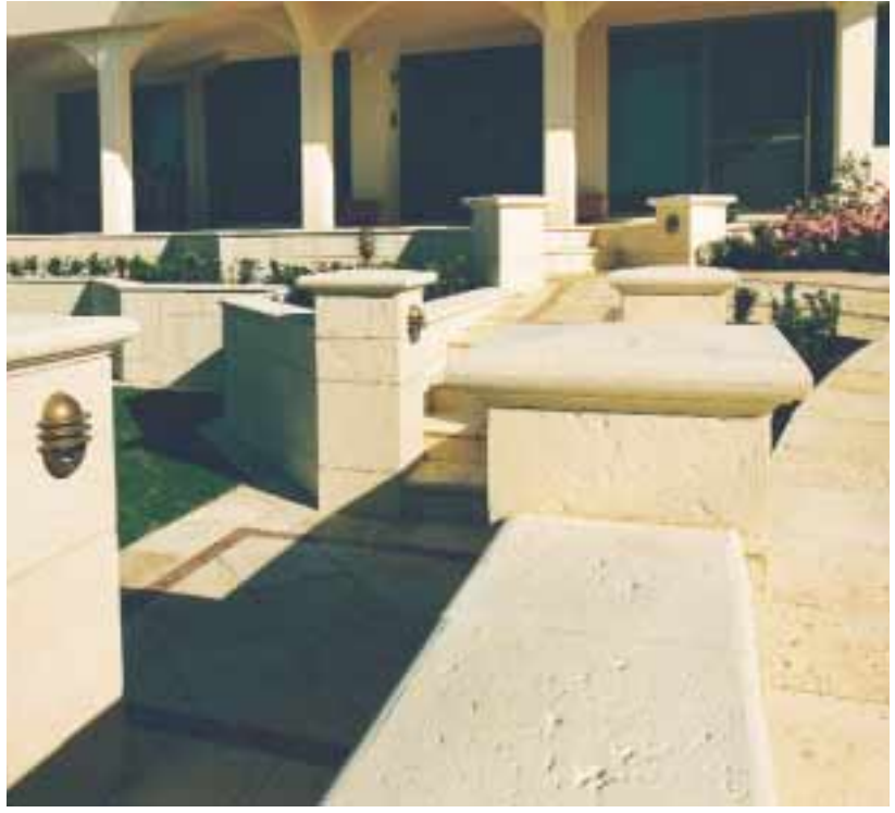
Limestone Reef cladding capped with single and double bullnoses.
