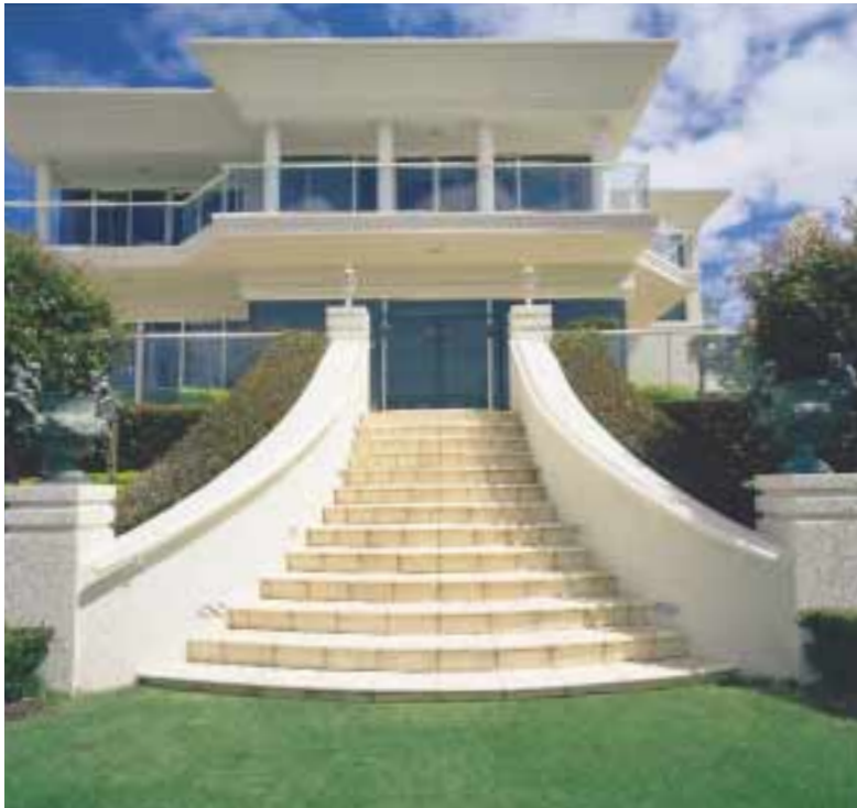
Limestone Reef cladding in a stair riser application, capped with single bullnose step treads.
